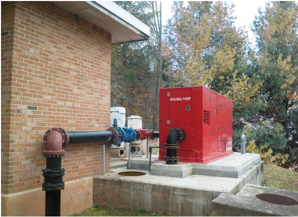
Being separate from both the duty electrical pumps and the electrical grid, Global Pump's independent engine-driven pump gives you the peace of mind that if something goes wrong, it is ready to go! Standard Sound Attenuated units reduce noise emissions to no more than 68 dBa at 30' (9 m). Varying dBa levels are available to meet design requirements.
